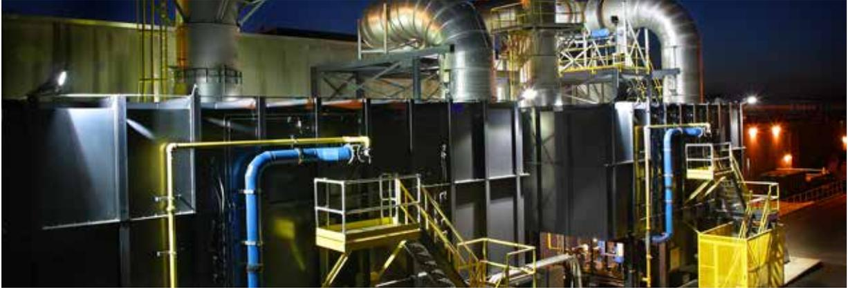
*Regenerative thermal oxidizers with switch valve*
