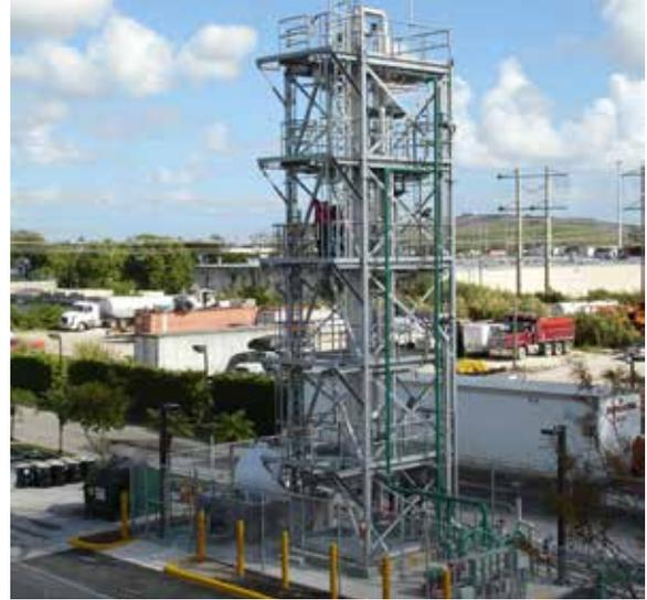
*Distillation system at pharmaceutical plant*
