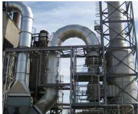
*Venturi scrubber on coal-fired boiler*
