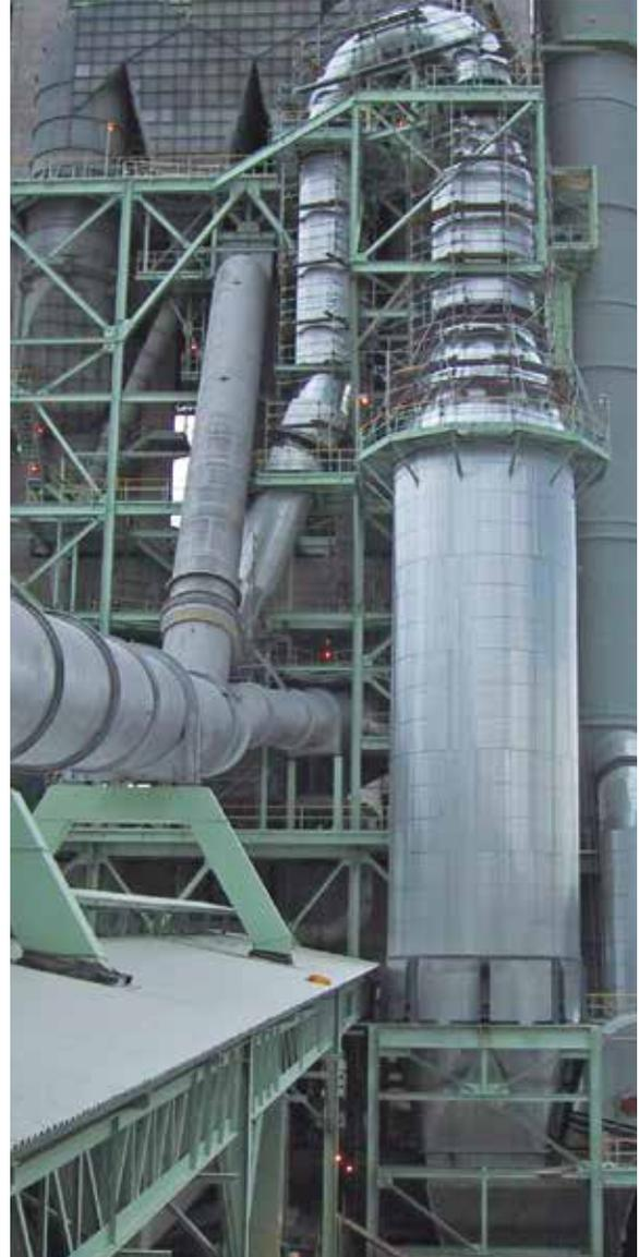
Evaporative gas cooling system in cement plant
