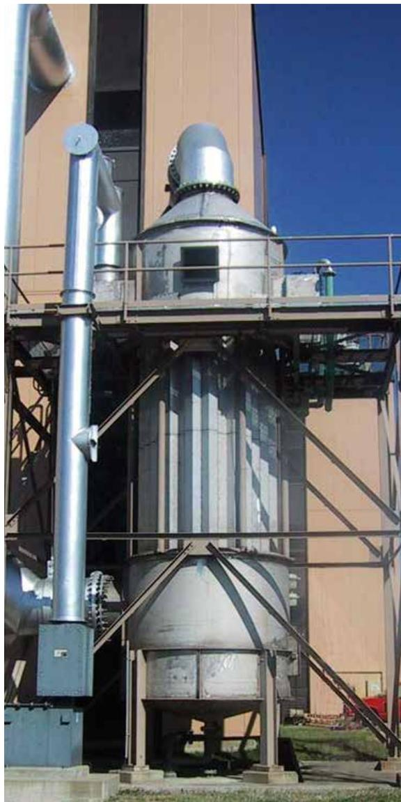
*Wet ESP for Hazardous Waste Combustion*
